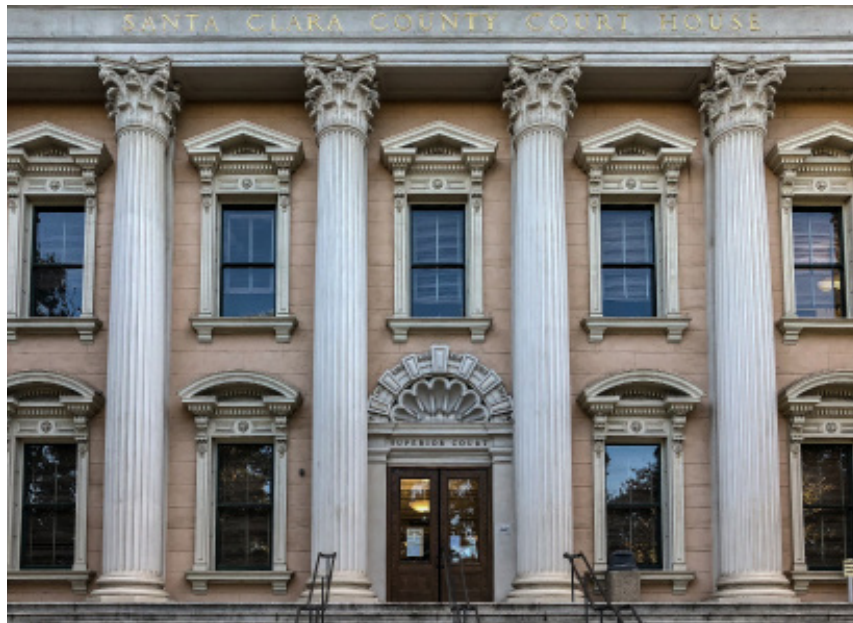
Historic Santa Clara County Superior Court House (Credit: Will Buckner)
